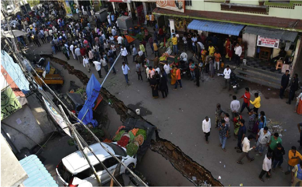
Fig. 4 Road stretch in Goshmahal, Hyderabad caved in due to Open drain/nullah covered by concrete slab below the road
