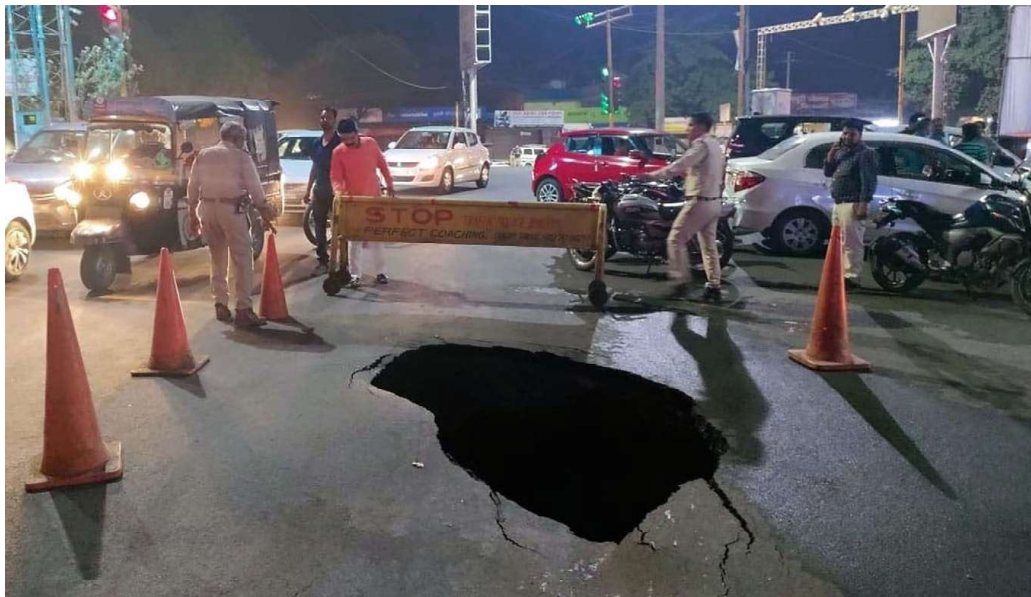
Fig. 3 A 10 feet sinkhole formed in Kolar area; Bhopal due to pipeline burst (01 May 2022)
