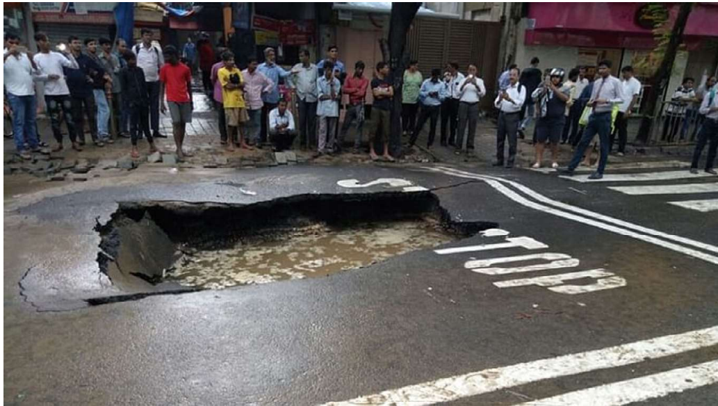
Fig. 1 Road caved in due to water pipe burst at Kalbadevi, Mumbai, Maharashtra (26 June 2018)
